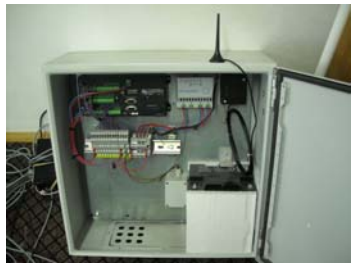
Fig. 4. The lockable steel cabinet
