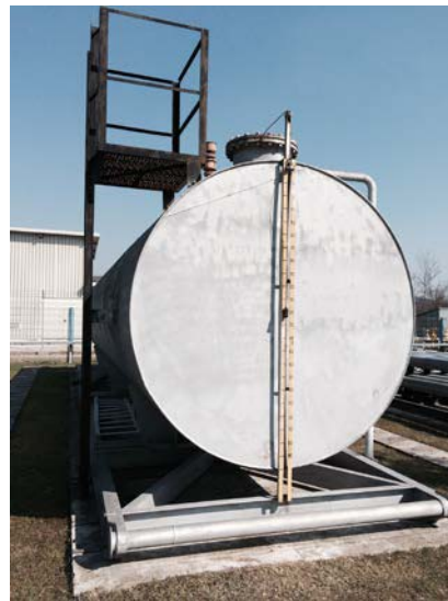
Fig 2. Horizontal reservoir / tank
